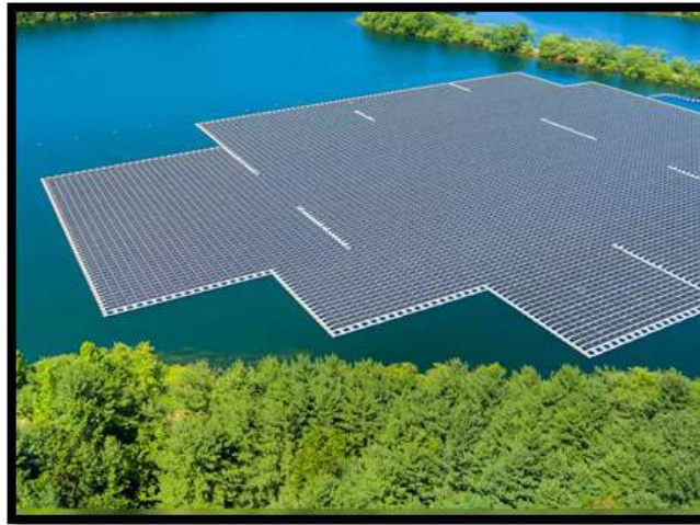
Floating Solar Panels, Image Source: (The Economic Times, 2023) at
