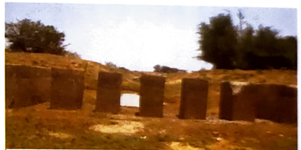
View of check dam in Jari GP under Binjharpur PS where catchment area is higher than the CD height
