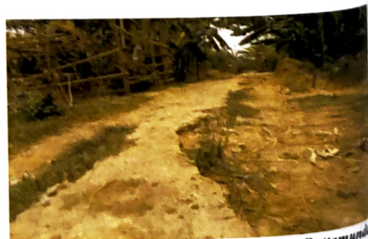
View of CC road in Beluria GP under Pattamunda PS damaged without cut off
