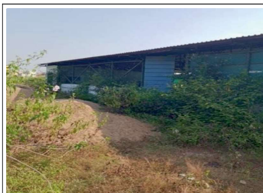
3.4.3(1) - Non-operational SLRM center at Chhatrapati Shivaji Ward, NPN Jagdalpur (Dt. 25.11.2022)
