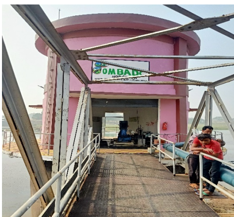
Picture-7: RCC structure intake well
