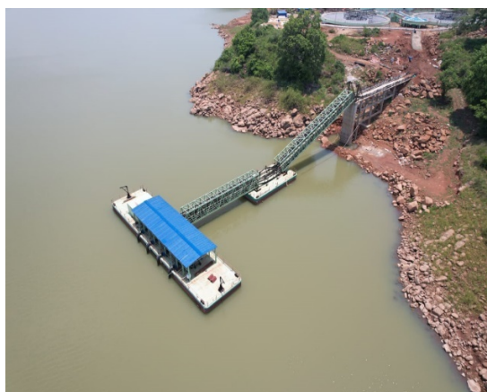
Picture-6: Floating jetty type intake well
