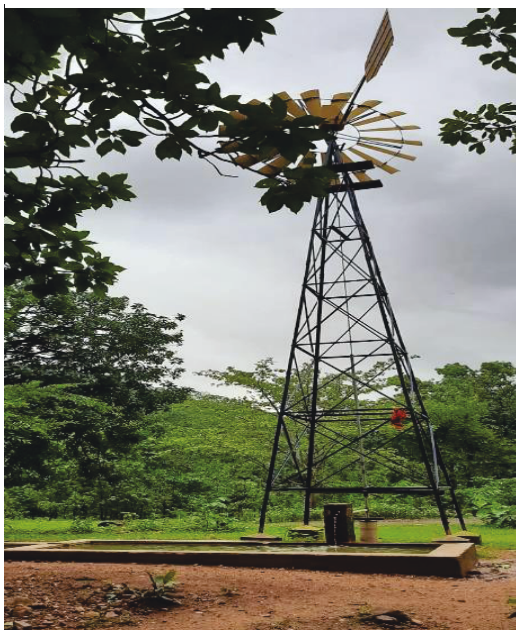
Photograph 4.5: Wind powered water pump (Jambughoda WLS)
