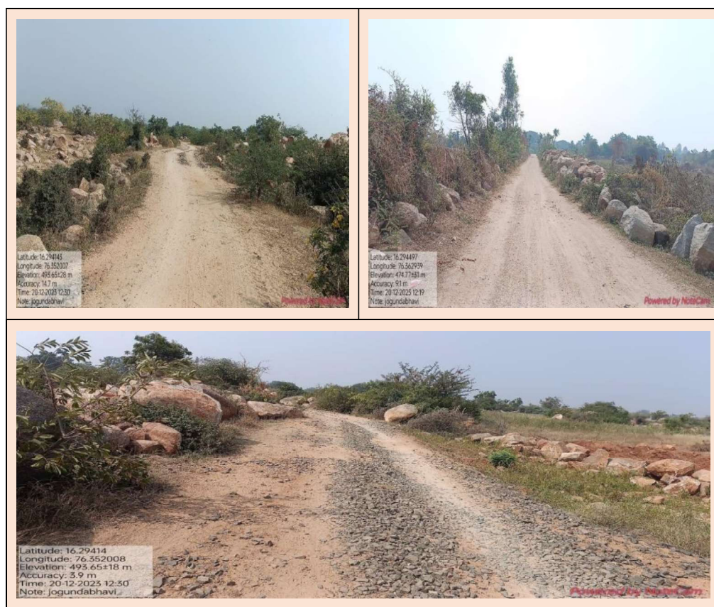
Picture No. 6.5.1: Photographs showing the status of road work
