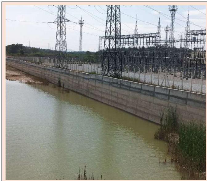
Picture No.6.6.2: Retaining wall view from tank side.
