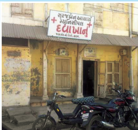
Picture 9 Dilapidated building of Municipal Dispensary in Bharuch NP
