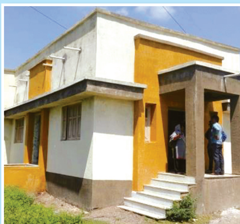
Picture 6 Community Hall at Fareni Road in Dhoraji NP lying idle since January 2015 for want of electricity and water connection
