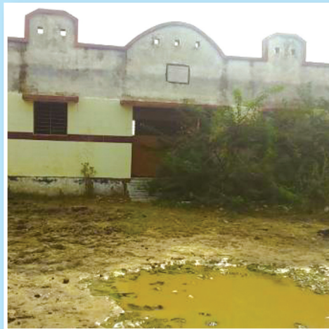
Picture 5 Pay and use toilet in Mehsana NP not being used for want of repair
