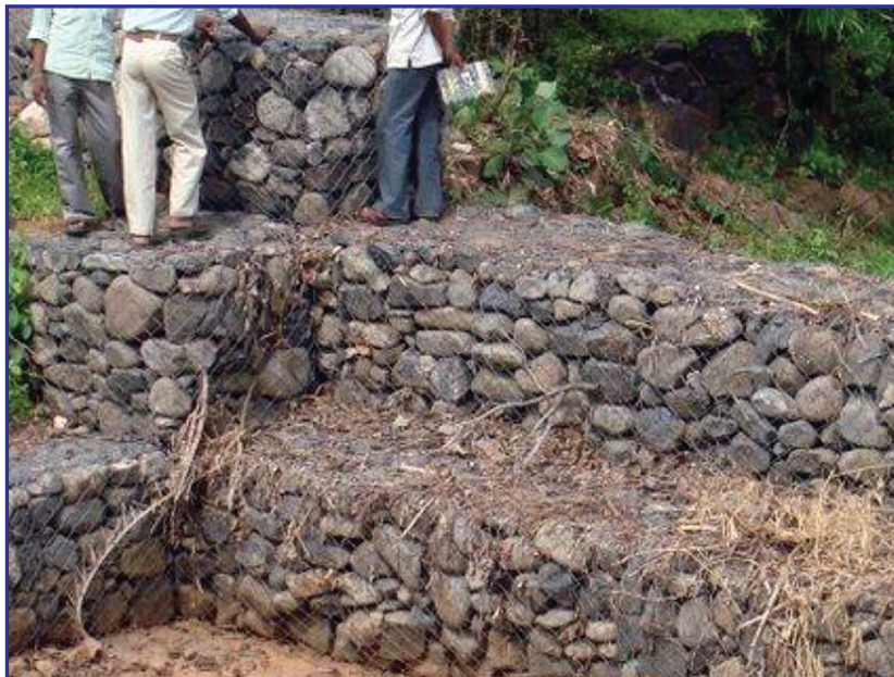
Picture 8 : Design of gabion structure (Technical Manual)
