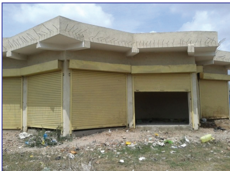
Picture 4: Renovated Zadeshwar village haat (02.07.2014)
