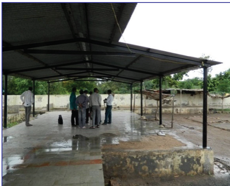
Picture 6 : Sayla village haat without separation wall and floor tiles coming apart (14.08.2014)
