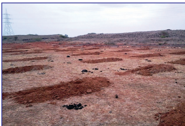
Picture 4 : Contour trench constructed in flat area in IWMP-4 of Kachchh (photo taken at the time of completion of construction work obtained from the records of DWDU)
