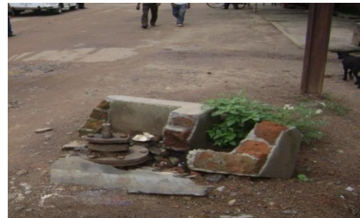
The sluice-valves are appearing above the road surface
