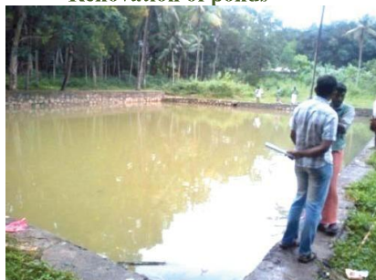
Renovation of ponds
