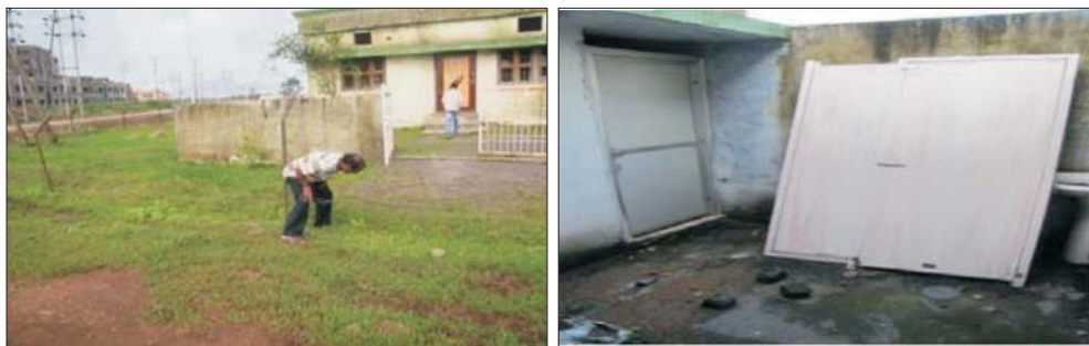
Photographs taken during joint physical verification on 3 August 2013 showing non-utilisation of the FIC at Ruabandha (Durg District)
