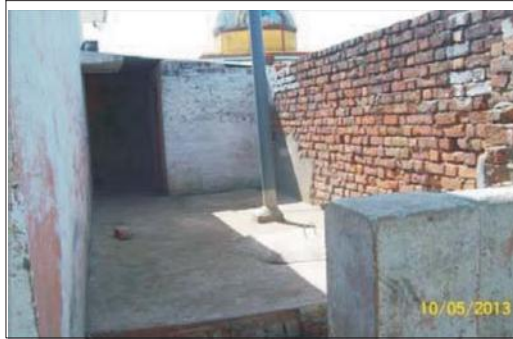
Photograph showing open bath room of Girl's Hostel at Nipania.
