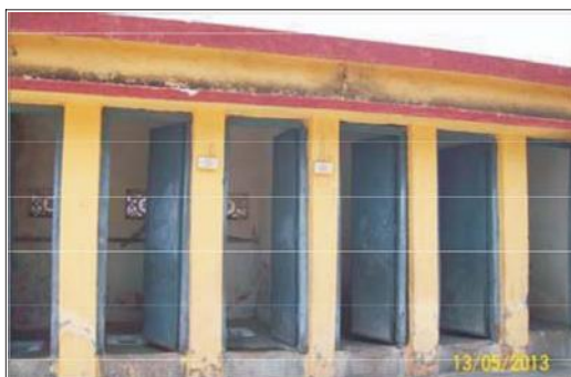
Photographs showing good condition of Toilets at Girls Ashram, Kasdol.
