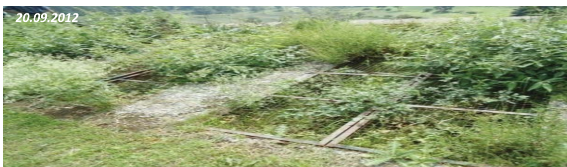
Unused composting pit at Narain Nagar, Nainital
