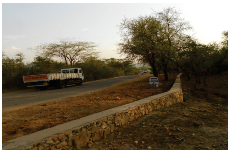
Traffic on SH 13 inside Sariska Wildlife Sanctuary
