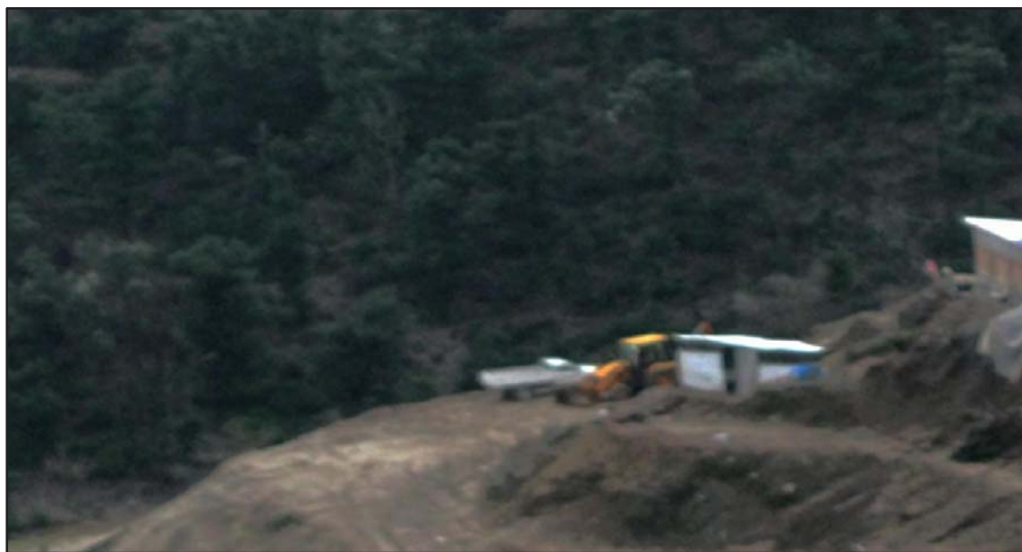
Gypsum mine Baryas in Assar, Doda
