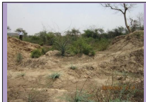
Dam constructed at village Ghamroj in Sohna Block washed away
