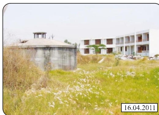
Overhead tank at Ground Level
