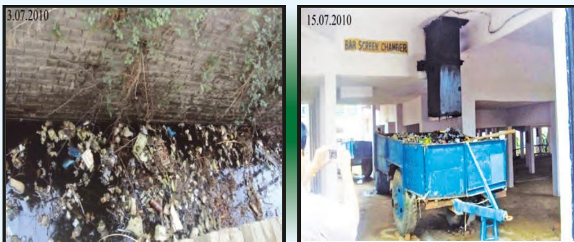
Choking of Gomtinagar drain due to plastic items and waste collected at STP, Daulatganj
