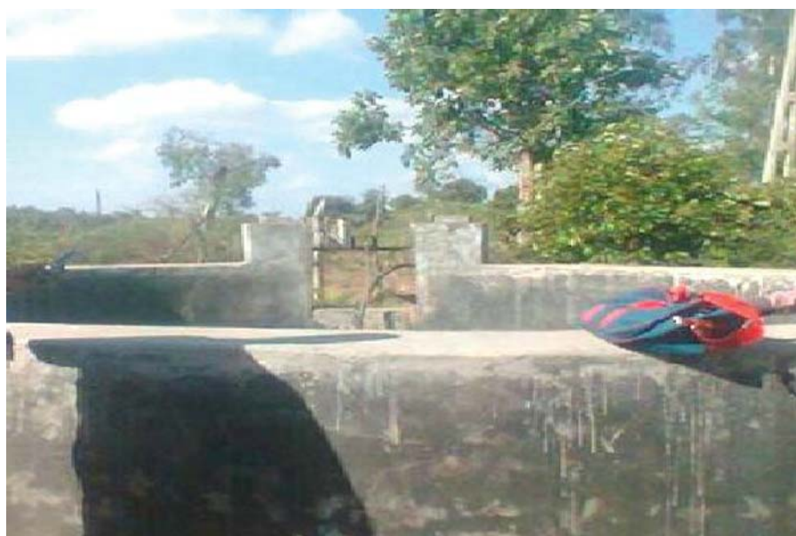
(Picture showing well with succession pipe, executed in private farm in Kakadkhila village – DWSC Dahod)
