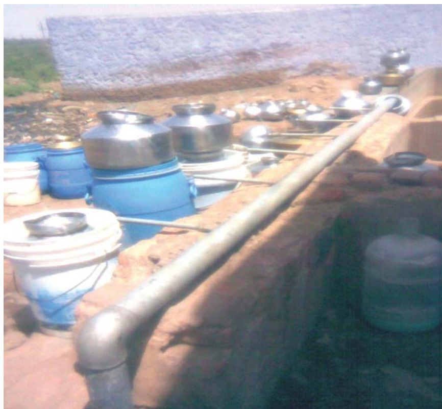
(Picture showing vessels kept in advance at stand-post by villagers of Hasanpur village)
