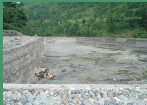
Incomplete MSWC production plant at Sipchu
