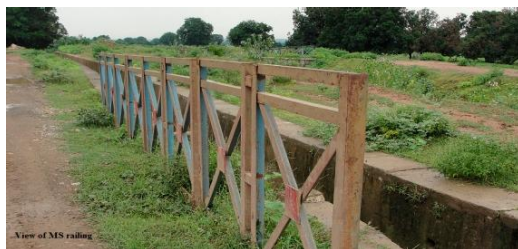
View of MS Railings
