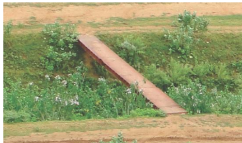
A mild steel footbridge installed over Sihawal canal
