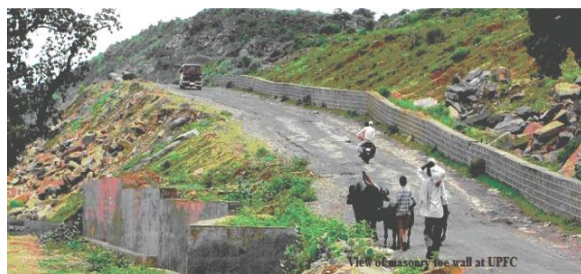
View of stone masonry toe wall of UPFC.
